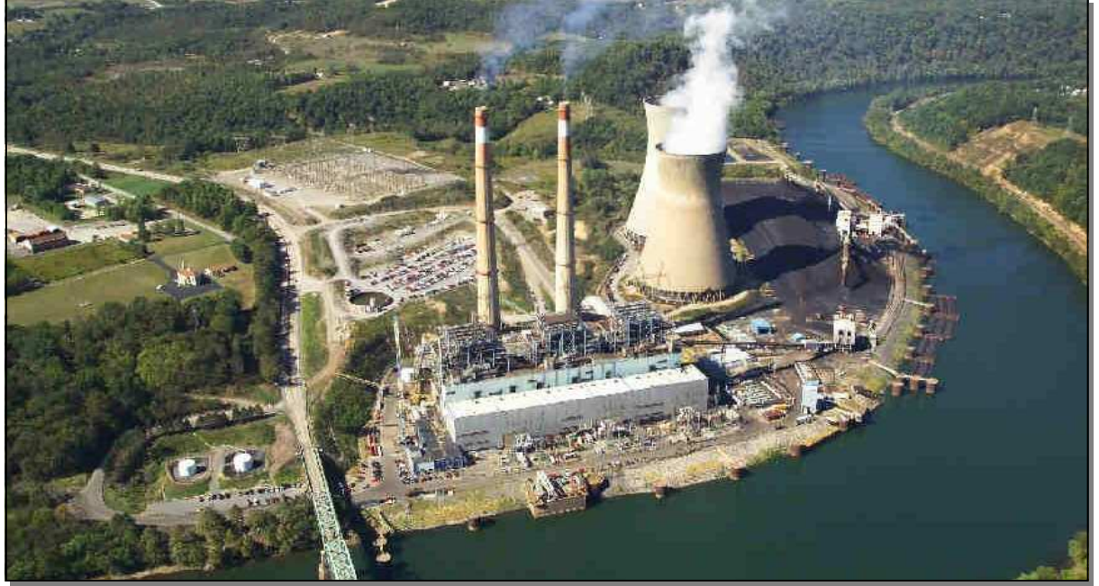
Hatfield's Ferry Power Station
