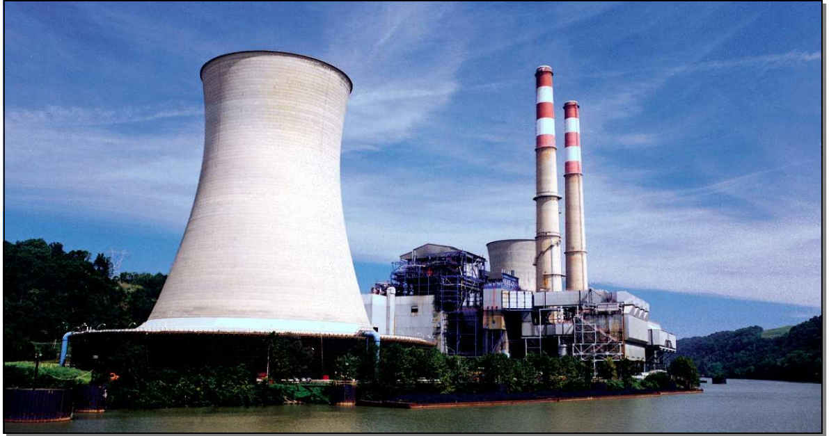
Fort Martin Power Station
